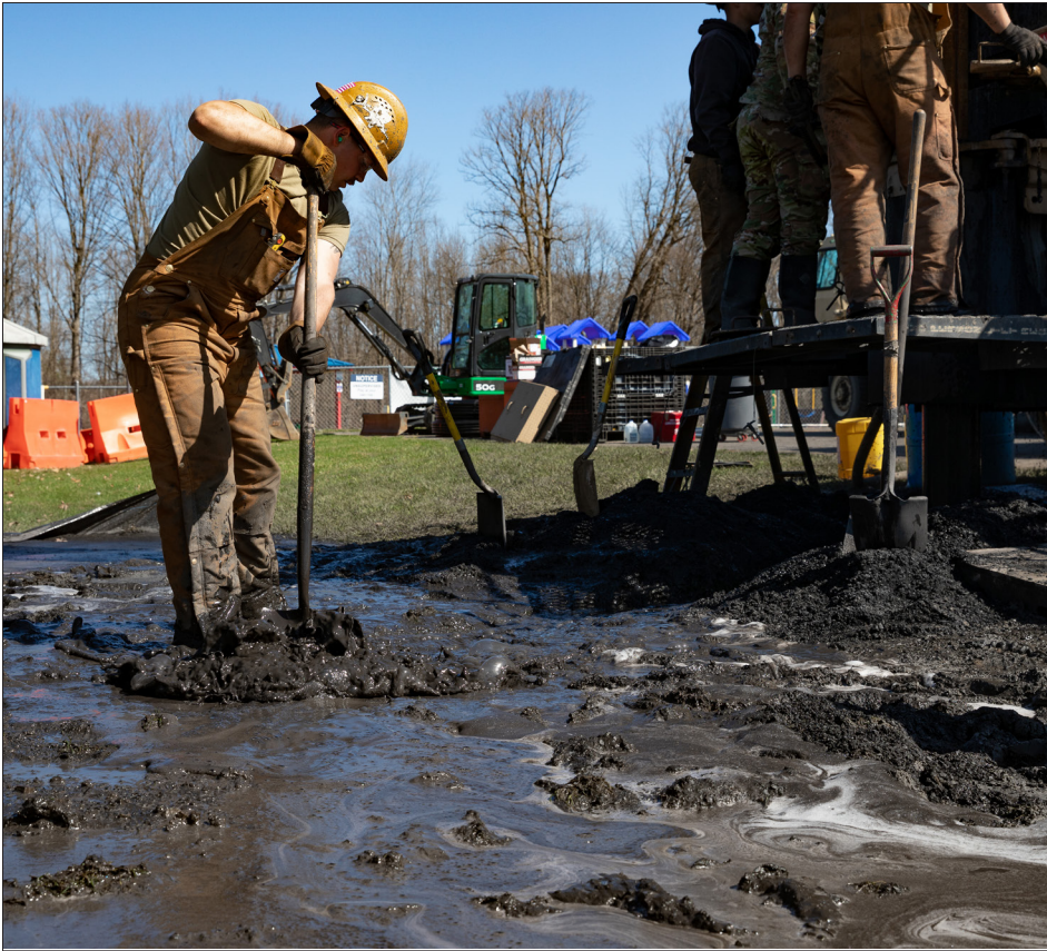
U.S. Army Spc. Brandon Turner, a horizontal construction engineer assigned to the 247th Engineer Detachment (Well Drilling), 192nd Engineer Battalion, Connecticut Army National Guard, clears a cut of debris at Naval Support Activity Saratoga Springs MWR, Saratoga Springs, New York, April 15th, 2022. Soldiers from the 247th drilled a well at the request of the U.S. Navy to support their Morale, Welfare and Recreation office, or MWR, during their annual training. (U.S. Army photo by Sgt. Matthew Lucibello)
