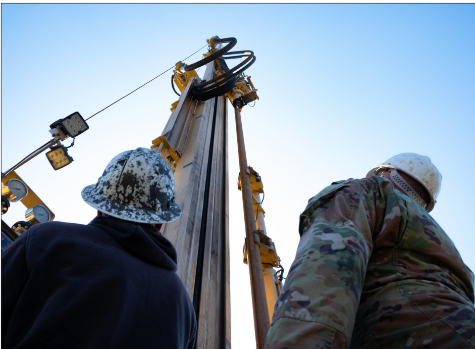
U.S. Army Spc. Denize Pine, left, and U.S. Army Spc. Donald Grande, right, horizontal construction engineers assigned to the 247th Engineer Detachment (Well Drilling), 192nd Engineer Battalion, Connecticut Army National Guard, observe the drill of a V-2000 drill rig at Naval Support Activity Saratoga Springs MWR, Saratoga Springs, New York, April 15th, 2022. Soldiers from the 247th drilled a well at the request of the U.S. Navy to support their Morale, Welfare and Recreation office, or MWR, during their annual training. (U.S. Army photo by Sgt. Matthew Lucibello)
